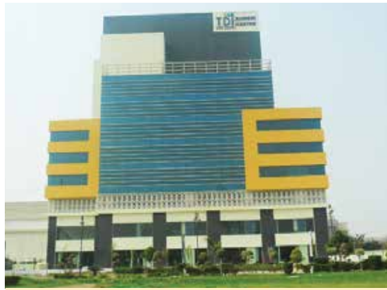
TDI BUSINESS CENTRE , MOHALI
